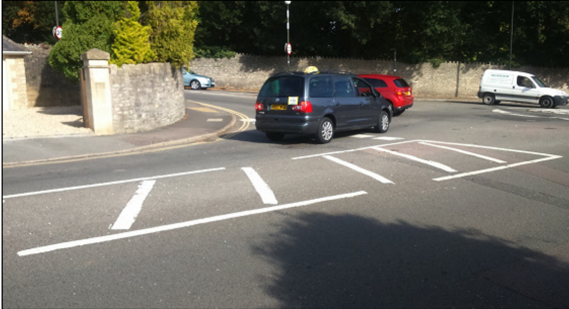
Existing one lane exit onto roundabout on Newbridge Hill
